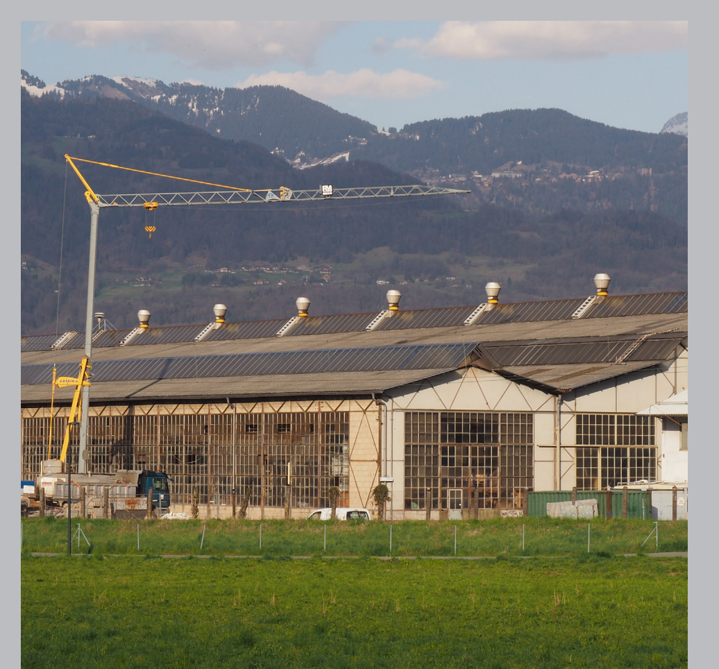
deconstruction of industrial sheds, providing corrugated metallic and transparent PVC plates
