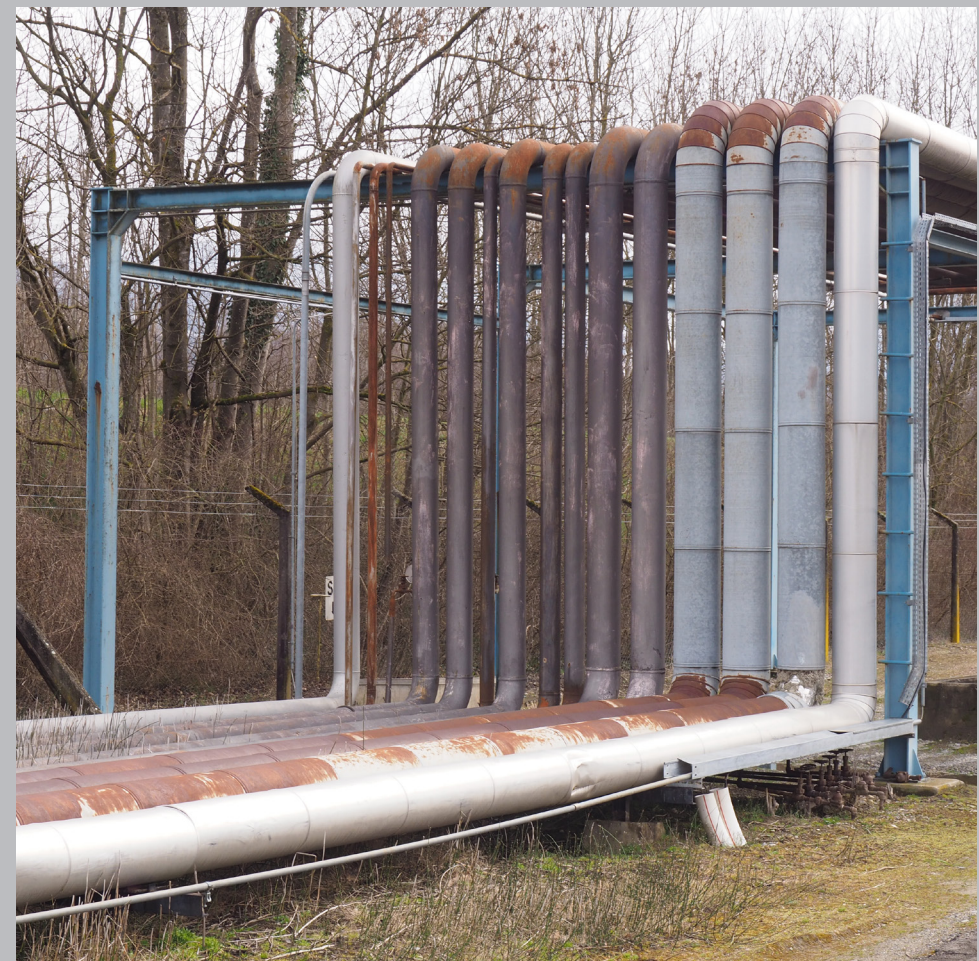
pipelines : 250 km of steel - 90 km pending dismantlement - preserved with azote
