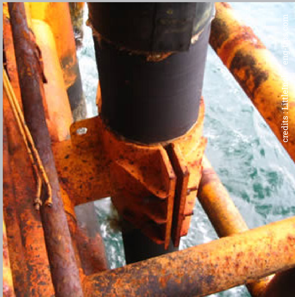
6 bolts oil platform clamp
