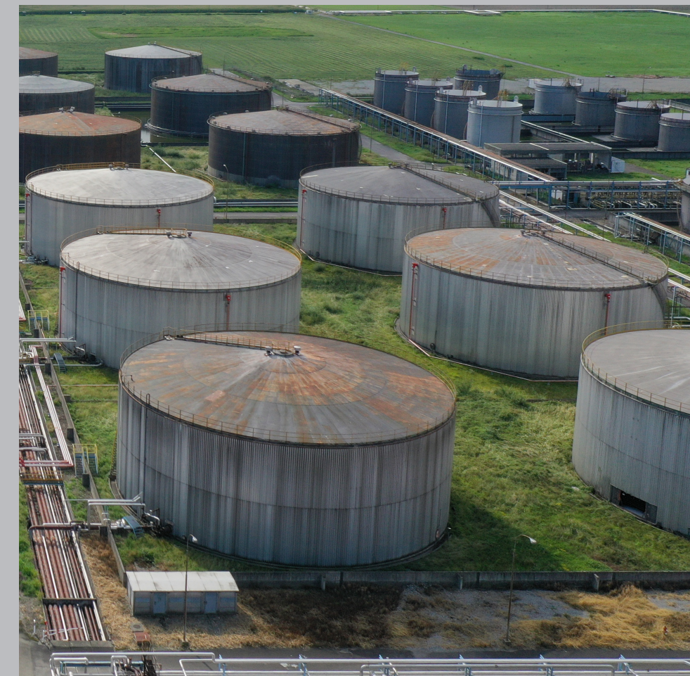
54 tanks - including some thermally insulated
