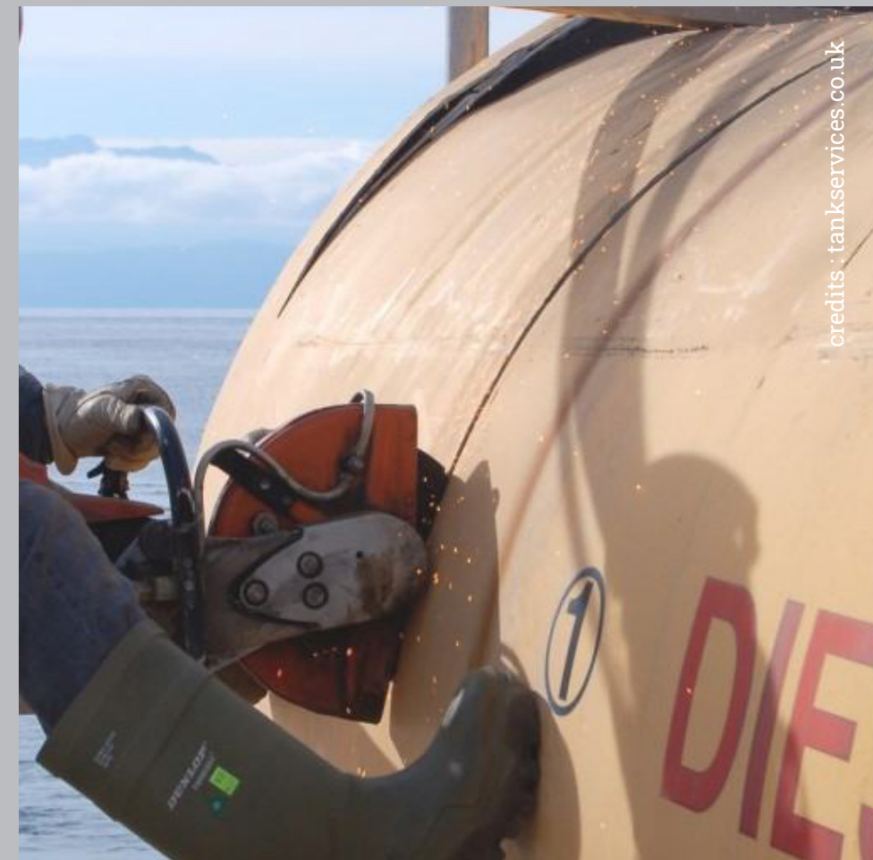
sawing only when needed and at maximum dimensions to minimize downcycling
