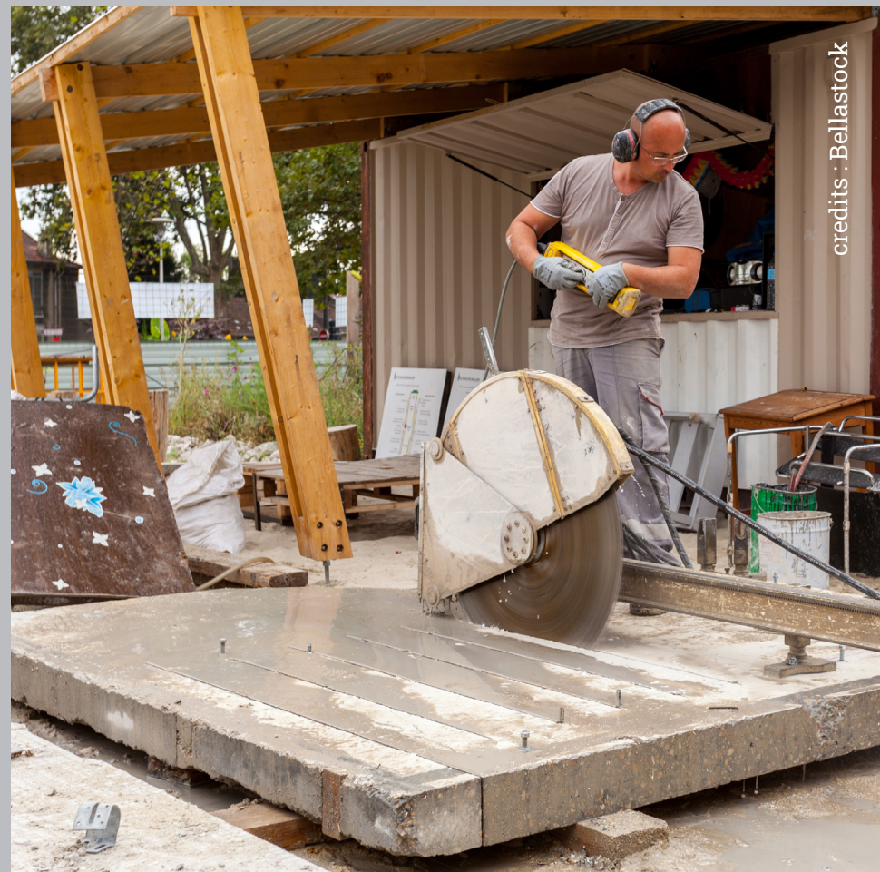
concrete "dismantlement" experiment using a diamond blade circular saw
